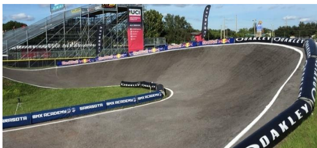
Good example of a second corner. Steep banking, and plenty of space to line-up before the third straight begins.
